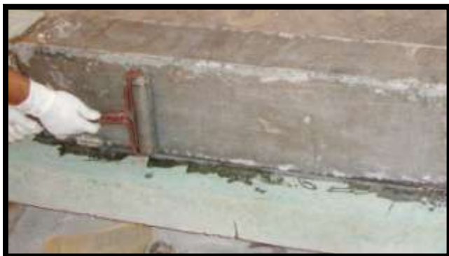
Fig 5: pressing to removal of air bubble
