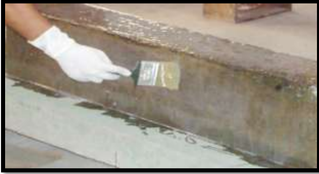
Fig. 3: Epoxy application on beam
