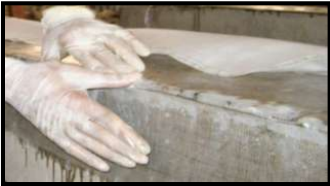
Fig 4: Fixing GFRP sheets
